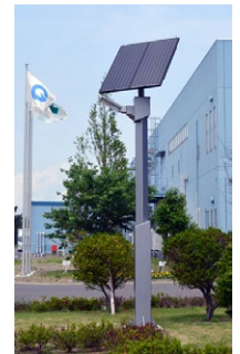
Solar-powered LED street lamp of the new building V-Wing of Goyo Electronics Co., Ltd.
