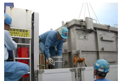
PCB-containing equipment being carried out
