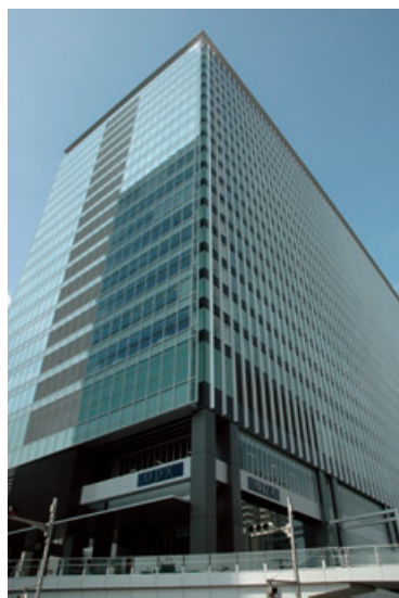
Head Office (Akihabara UDX Building, 11th floor)
