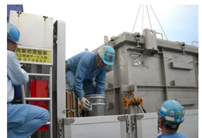
PCB-containing equipment being carried out
