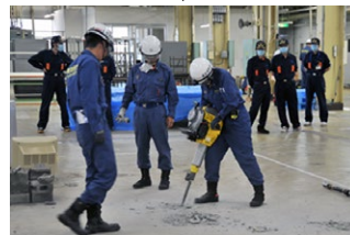
Practice of drilling a hole on a concrete floor
