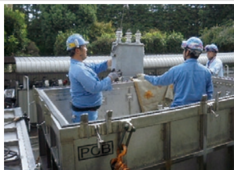
PCB-containing equipment being carried out
