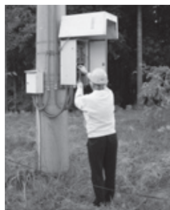
Disaster prevention radio units being inspected one after another immediately after the disaster
