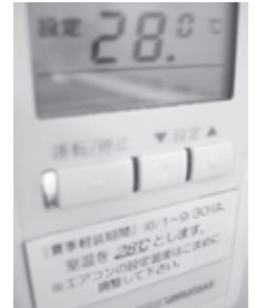
Display of air-conditioner's setting
