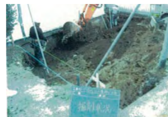
Replacement of soil
