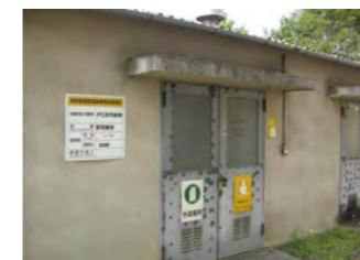
PCB storage warehouse
