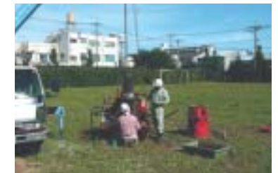
Sample collecting for soil investigation
