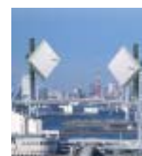
● Wireless Broad Band System Network established with micro waves where cable cannot be used such as across rivers, public roads, and places between buildings.
